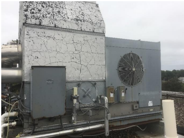
Cooling Tower — Galvanized — Outdoor Unit
