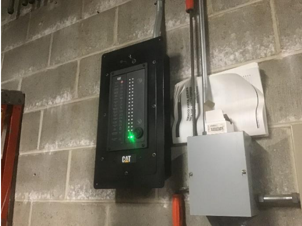
Emergency Generator Transfer Switch
