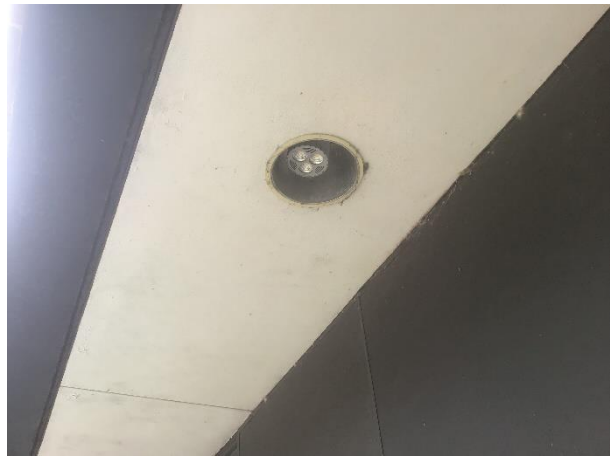
Exterior Recessed Can Light Fixtures
