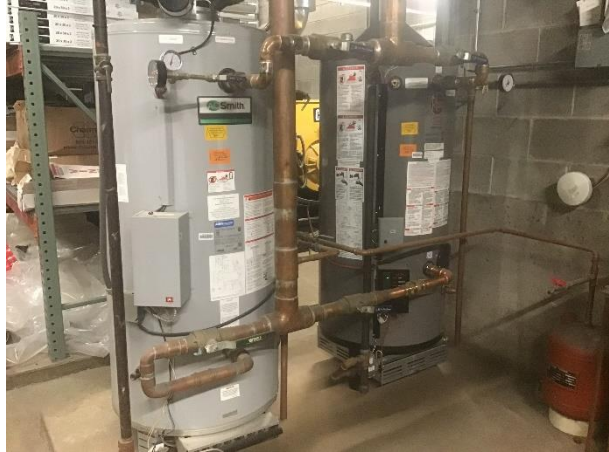
Domestic Hot Water Heater — Gas
