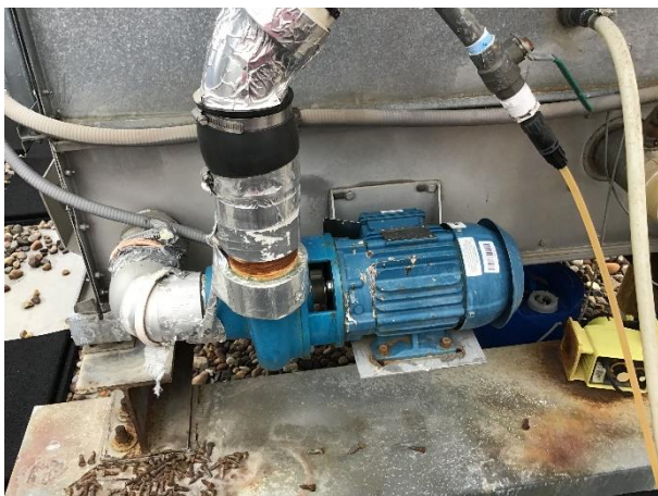
CW Circulation Pump and Motor, 0.5 to 1 HP
