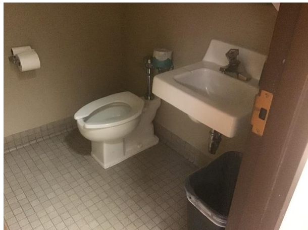
Floor Mounted Water Closets
