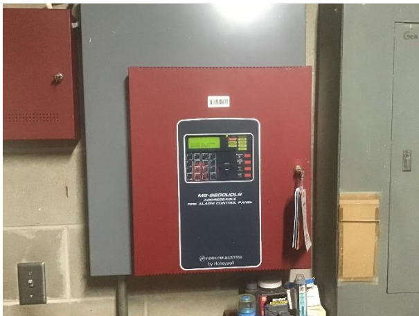
Fire Alarm Control Panel, FACP, Up to 10 Zone
