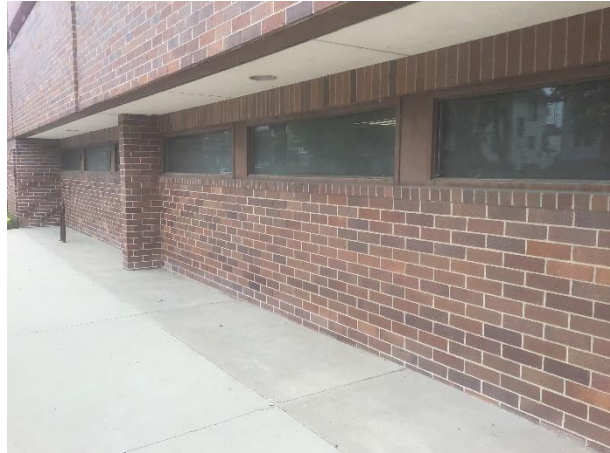
Aluminum Window Units — Fixed or Single Hung
