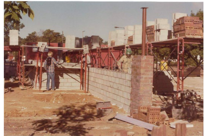
Masonry (CMU) foundation construction
