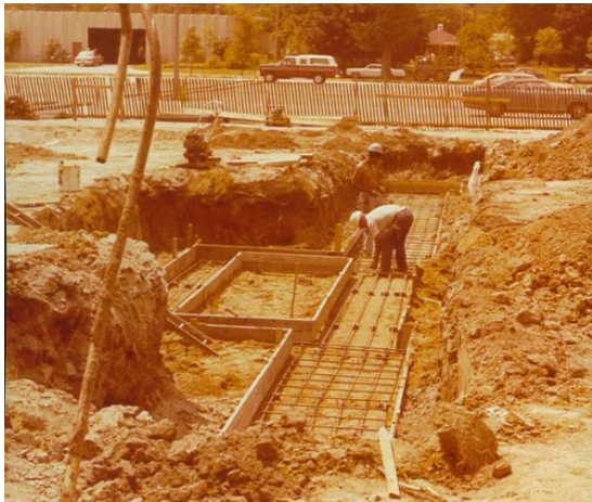
1979 photo of footing construction
