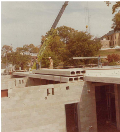
Hollowcore precast second level floor construction
