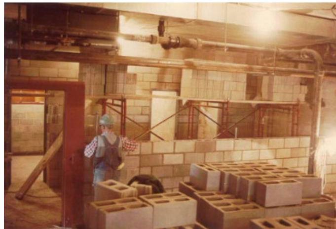
Masonry (CMU) construction of interior walls
