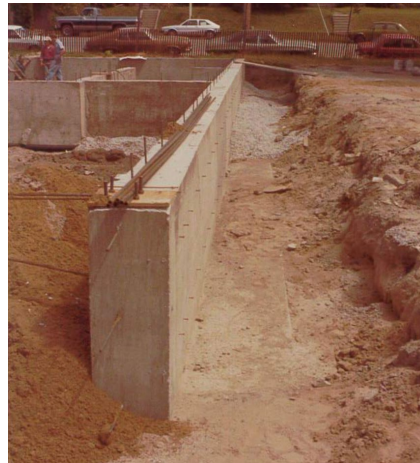
CIP PCC foundation and footing
