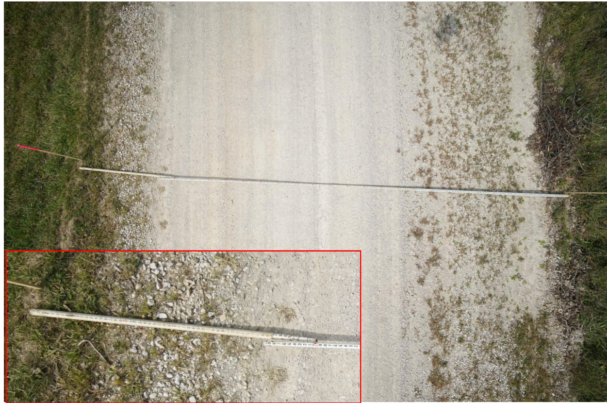
LOCATION 3 CLOSE VIEW
