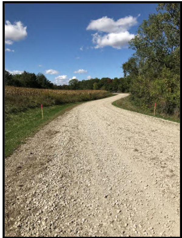
Gravel Base Width Between Stakes – 24' (28' total between stakes)
