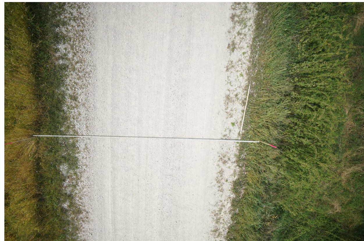
LOCATION 4 CLOSE VIEW
