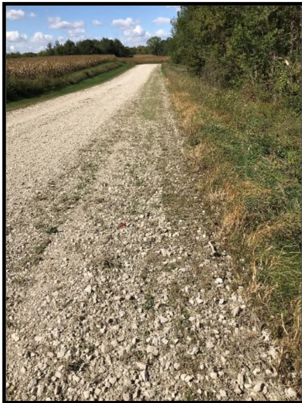
Uncovered Rock Base After Grading – 7'
