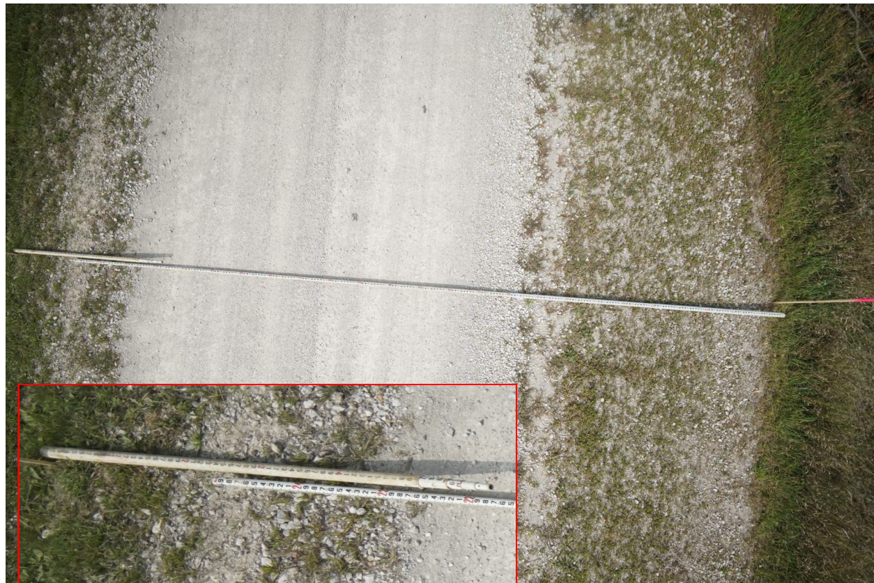
LOCATION 2 CLOSE VIEW
