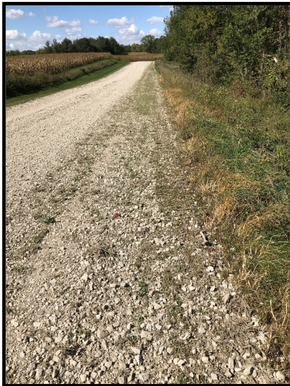
Uncovered Rock Base After Grading – 7’
