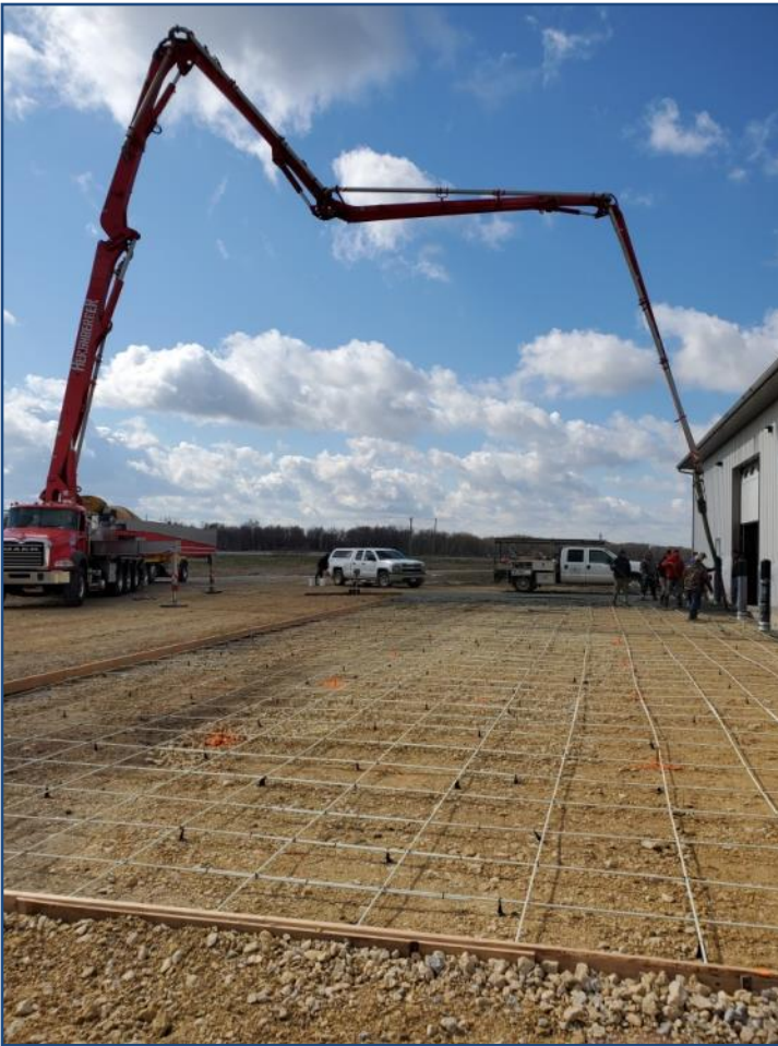
Staff excavated, formed, helped pour and finish the concrete apron accessing the east side of the building and bay doors.
