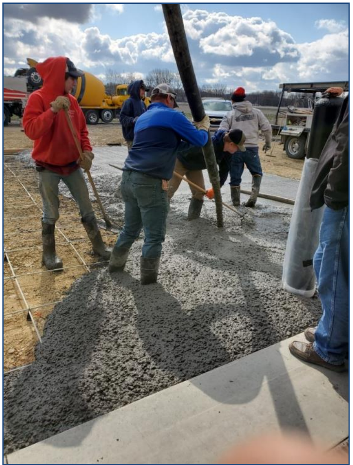
Staff excavated, formed, helped pour and finish the concrete apron accessing the east side of the building and bay doors.
