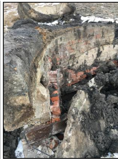
An old well used to provide water to the barn in the 1930's was abandoned years ago. Located on a natural wetland seep, the well was contaminated with surface runoff. The well lining was removed, filled with bentonite and site restored to its native condition for restoration of a wetland seep plant community.
