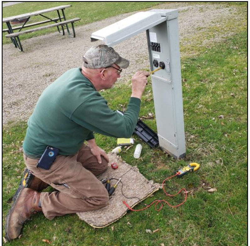
Dave Gustafson, Utility Person, repairs an electrical pedestal in the campground. Maintaining the electrical system and inspecting campground service pedestals at Kent Park and Hill's Access Campground requires continual attention. Each time Hills Access Campground floods the entire electrical system is shut down, inspected, cleaned and then re-energized.
