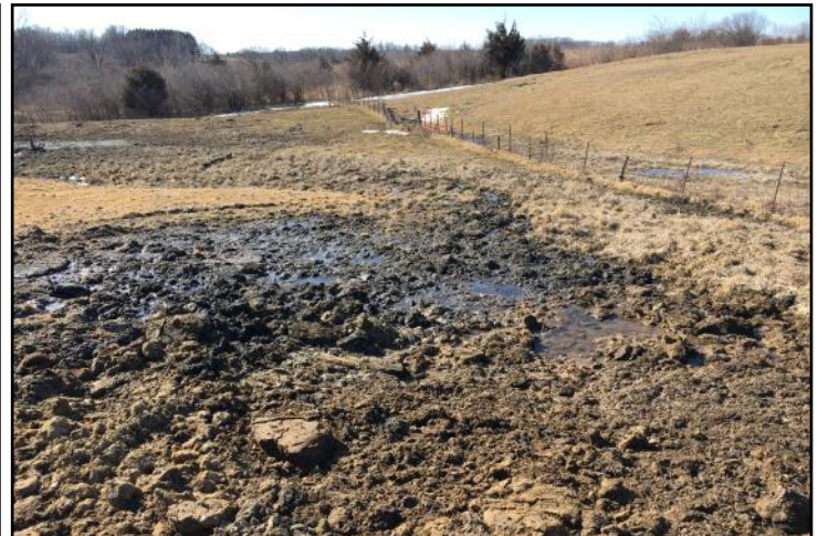
An old well used to provide water to the barn in the 1930's was abandoned years ago. Located on a natural wetland seep, the well was contaminated with surface runoff. The well lining was removed, filled with bentonite and site restored to its native condition for restoration of a wetland seep plant community.
