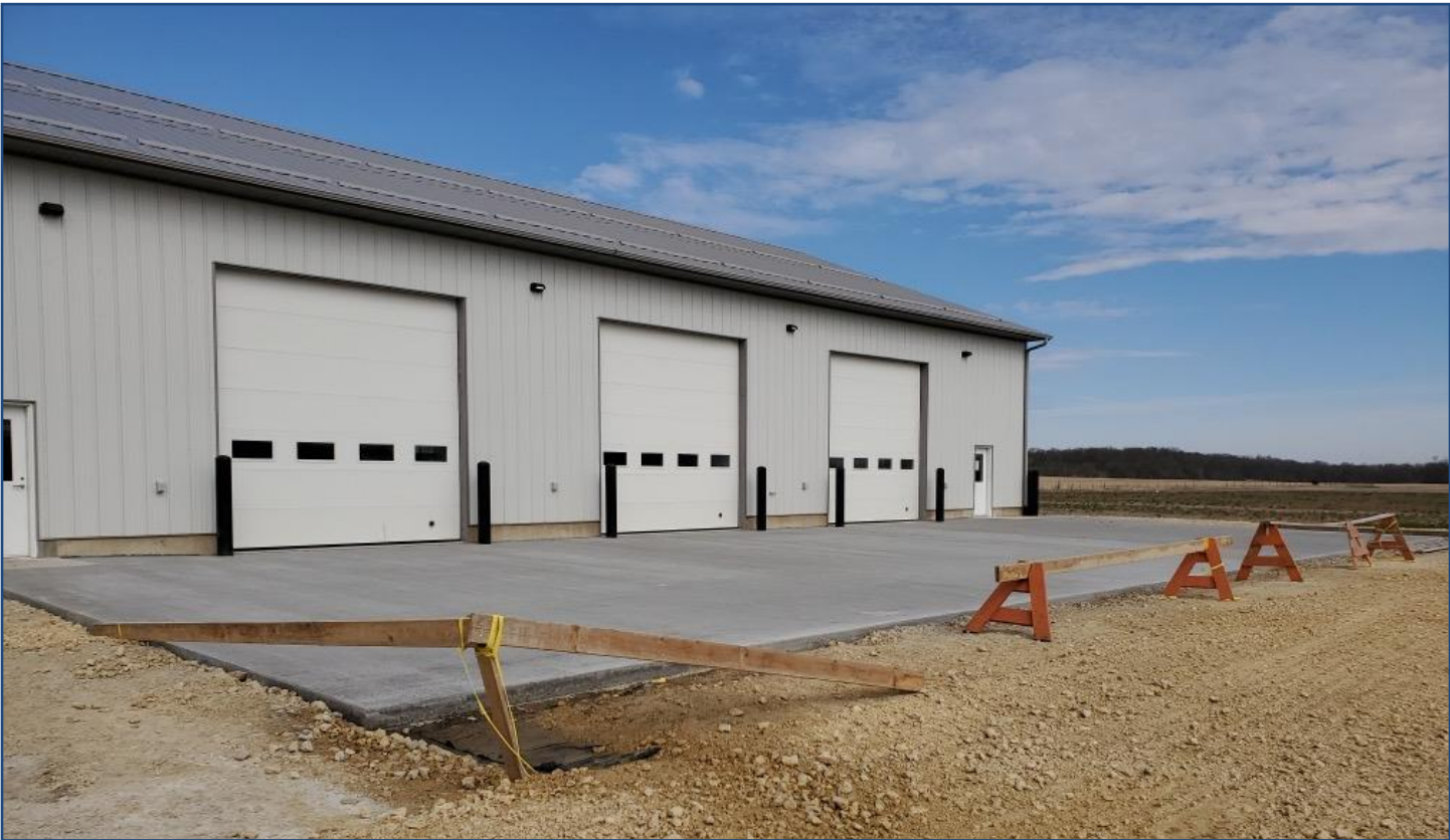
Staff excavated, formed, helped pour and finish the concrete apron accessing the east side of the building and bay doors.
