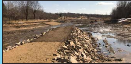
Four submerged fish reefs will include spawning beds. The aquatic plants will be planted on the surface of the reefs.
