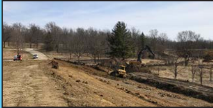
Connolly Construction Inc. employees grade the backslope of the dam in preparation for the prairie seeding.
