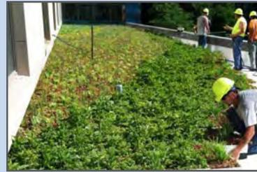
**WHAT IS GREEN INFRASTRUCTURE?** Green infrastructure utilizes natural vegetation to capture, store, and infiltrate stormwater runoff such as bioswales (large water collector), rain gardens (small water collector), and green roofs pictured above. It provides a range of critical functions and ecosystem services to communities, such as wildlife habitat, stormwater management, and recreational opportunities.\*
