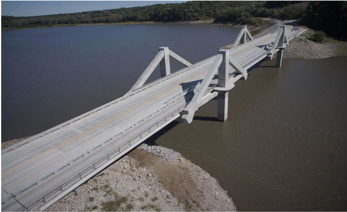
Mehaffey Bridge (completed October 2015)
