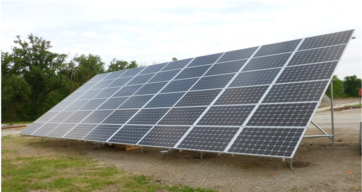
Solar Array at Secondary Roads Building
